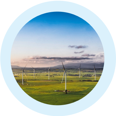
Stockyard Hill Wind Farm
